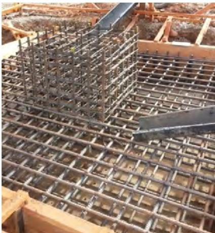
Thickener Center Column footing before concrete pouring.
