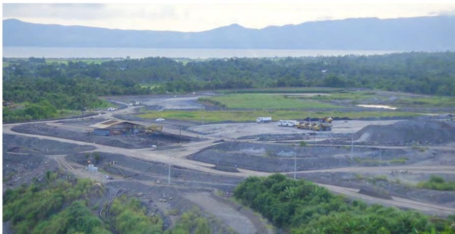
Overview of TSF3 with left edge showing completed rock-fill blanket on tailings beach. The trucks are parked on the RoM pad extension while waiting for a blast in the open pit.
