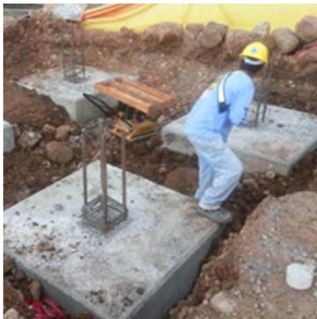
Stair Tower footing after concrete pouring.
