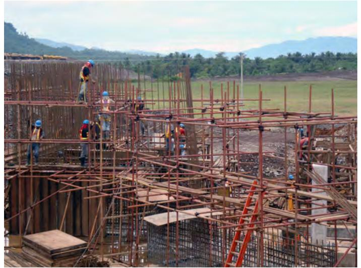
Rebar and formwork preparation for concrete pour of back retaining wall of crusher station.
