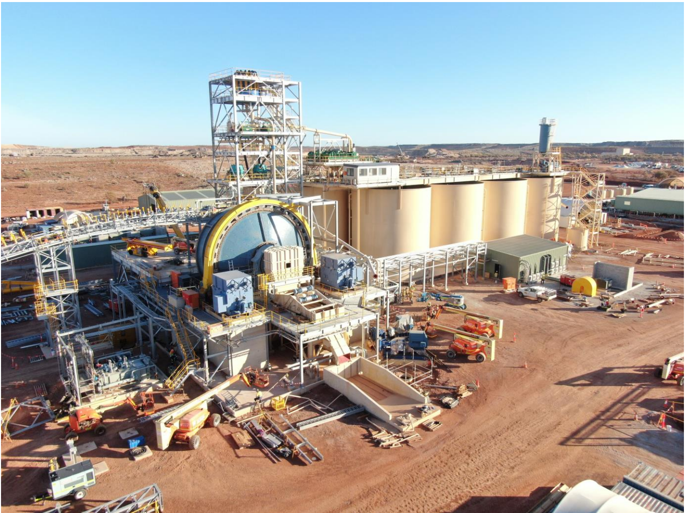
Figure 2: Construction of the KOTH SAG Mill as at 20 January 2022.
