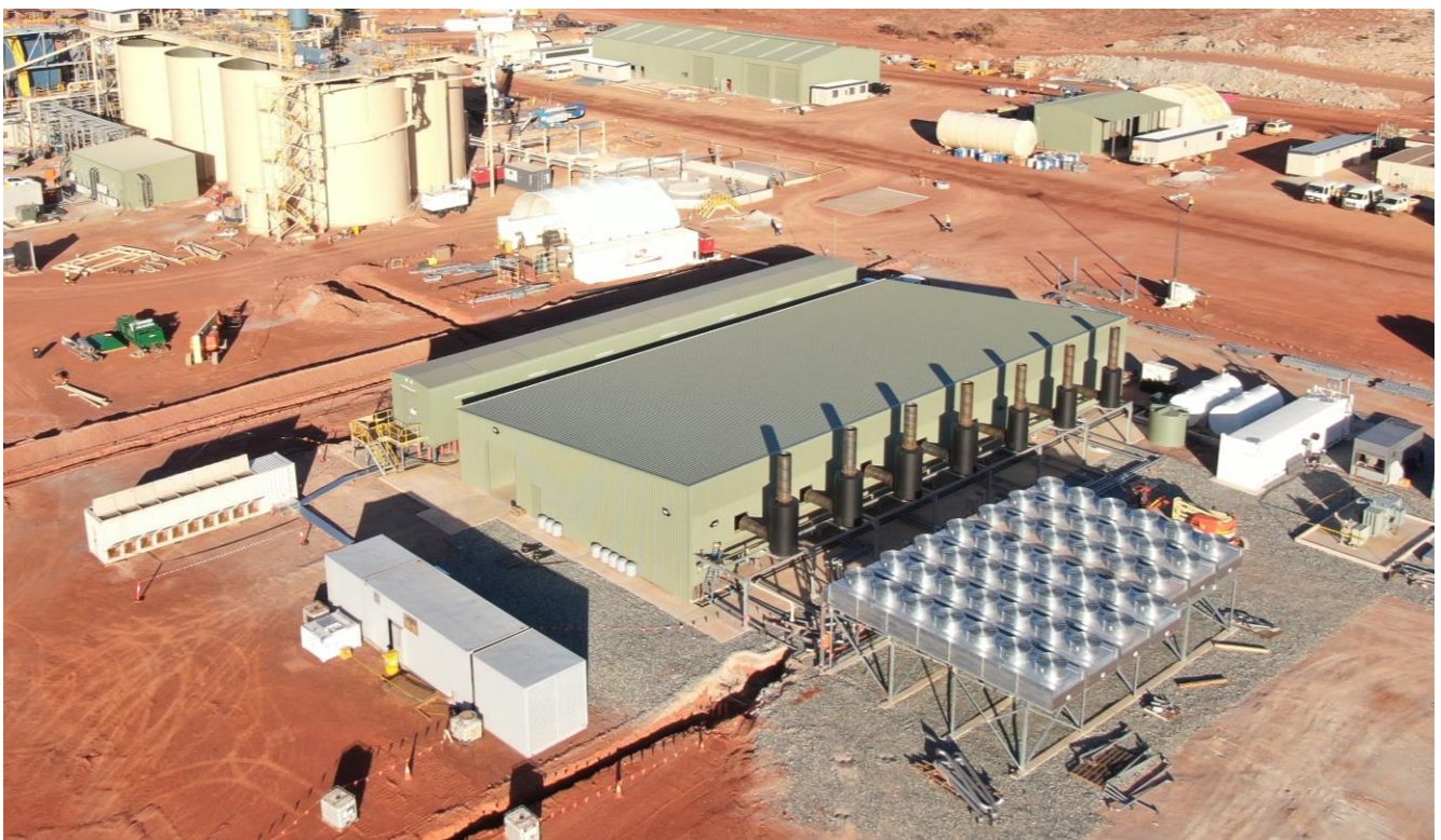
Figure 4: Construction of the power station as at 20 January 2022.
