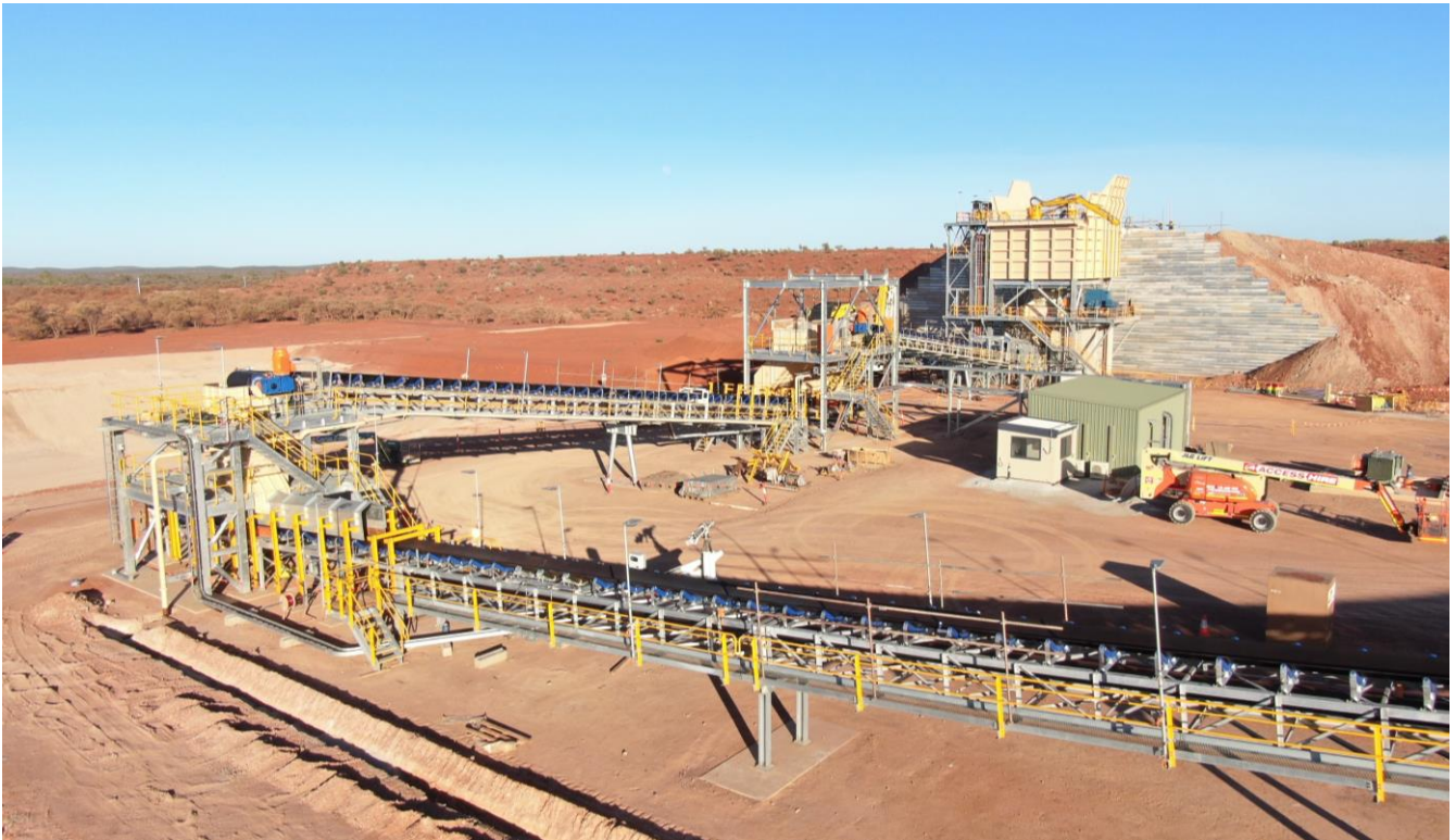
Figure 3: Construction of the KOTH gyratory crusher as at 20 January 2022.
