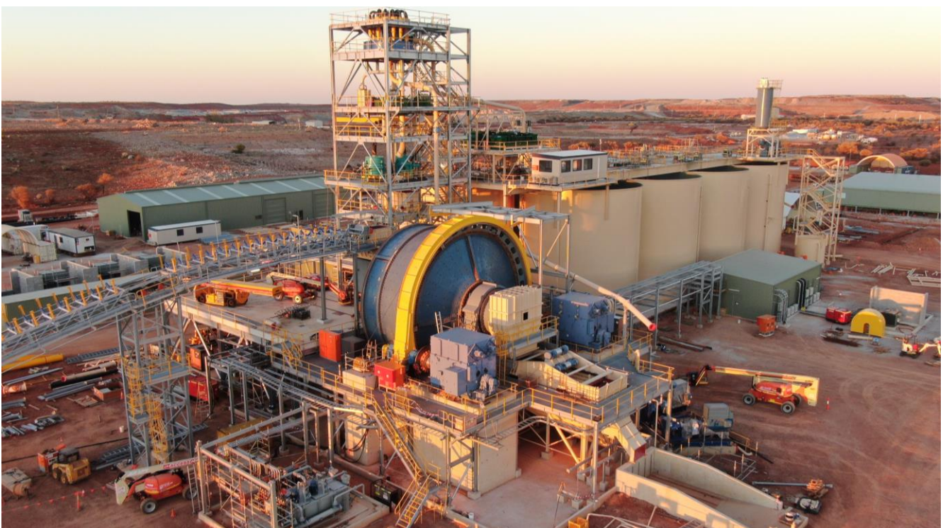
Figure 3: Construction of the KOTH SAG Mill as at 21 January 2022.
