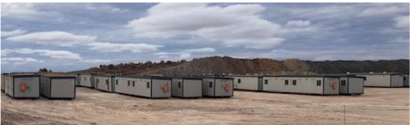
Figure 23 Second-hand camp modules delivered to KOTH, ready for installation.
