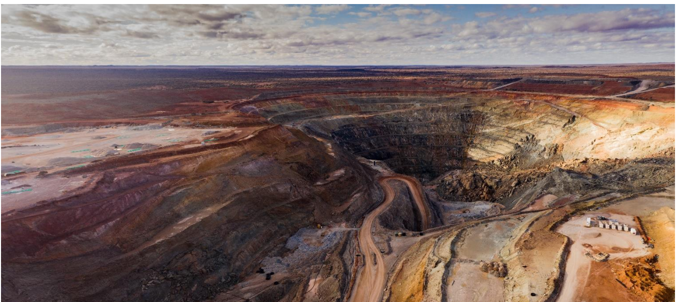
Figure 14 North Pit with historic eastern wall failure visible (the area is not mined until 2027).
