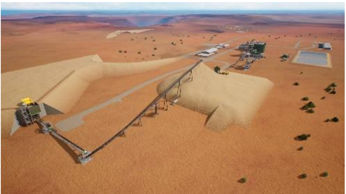
Figure 21 Artist impression of planned crusher, CIL plant and infrastructure, KOTH open pit.
