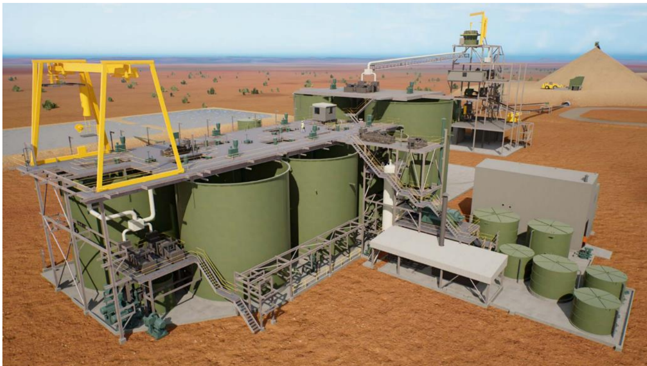
Figure 6 Artist's impression of the planned 4Mtpa CIL plant at King of the Hills.
