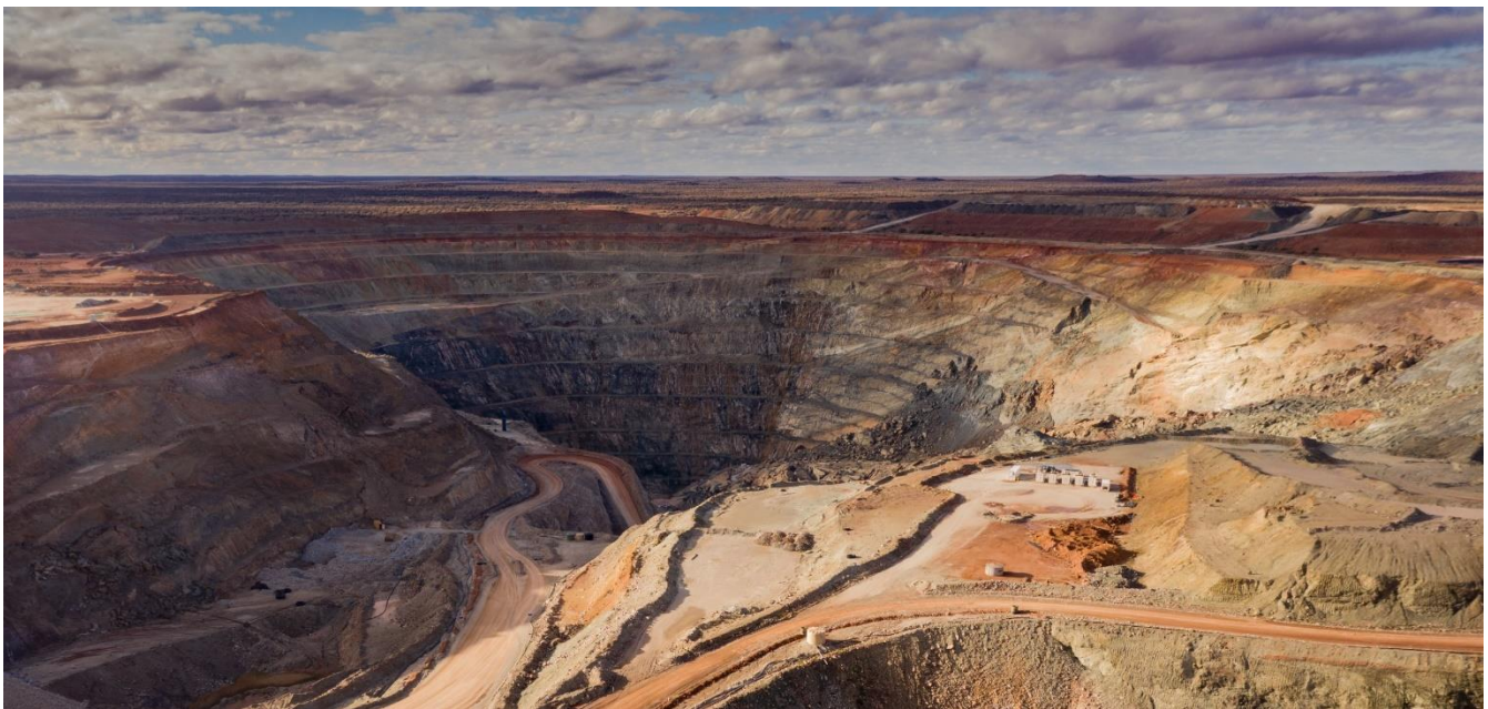
Figure 1 KOTH North Pit with access to the underground portal.
